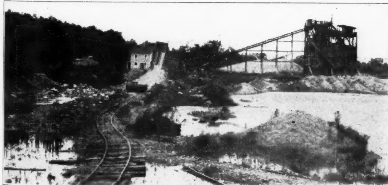
General View of Iron Ledge Company's Sand and Gravel Plant.
